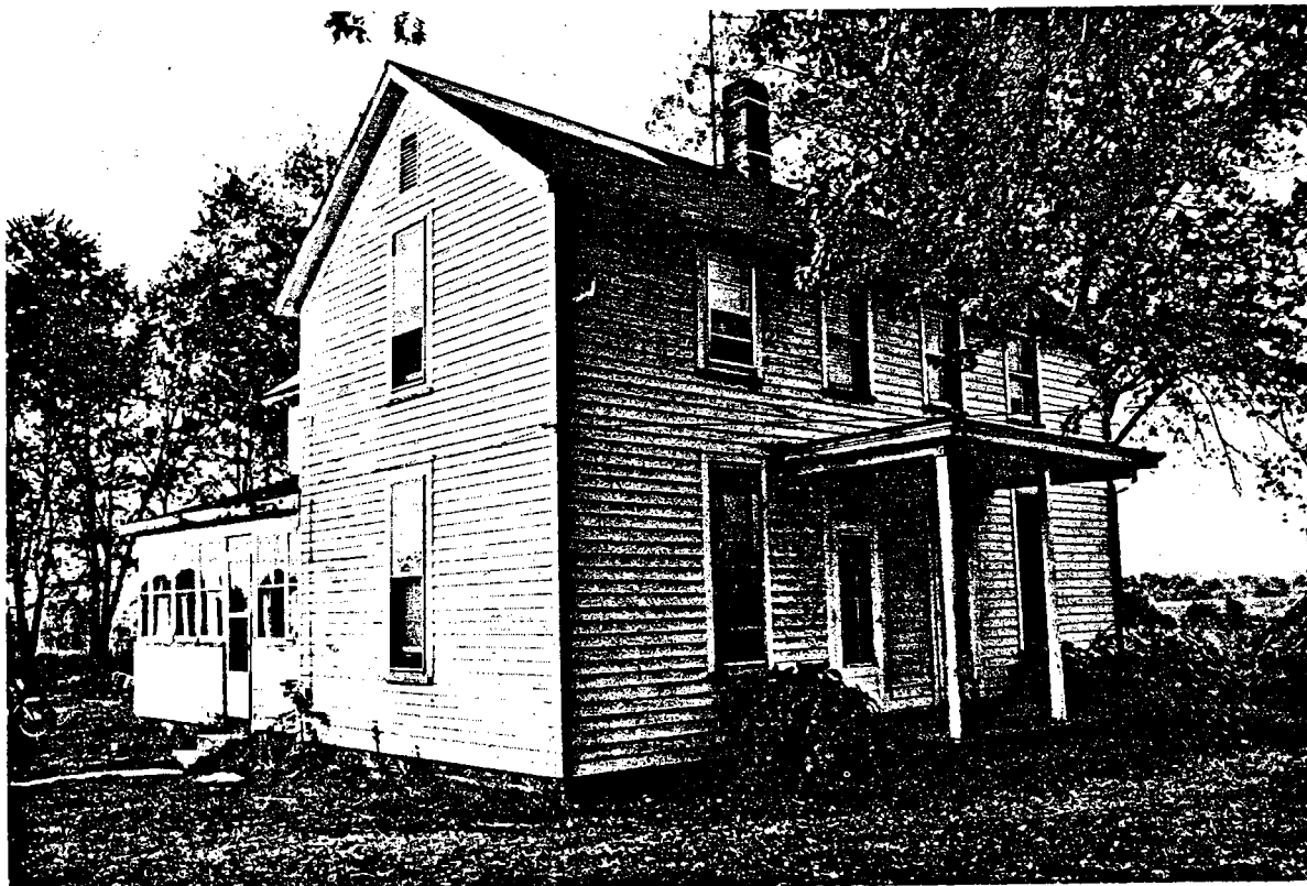
Figure 15.—Test structure 19, near a coal mine.
