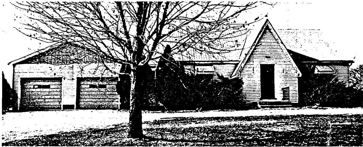
Figure 16.—Test structure 20, near a coal mine.
