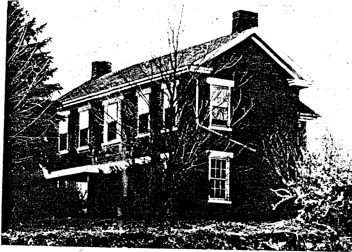
Figure 27.—Test structure 51, near a coal mine.
