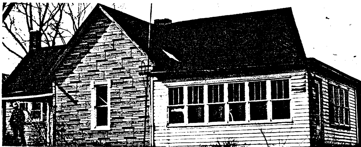
Figure 21.—Test structure 27, near a coal mine.
