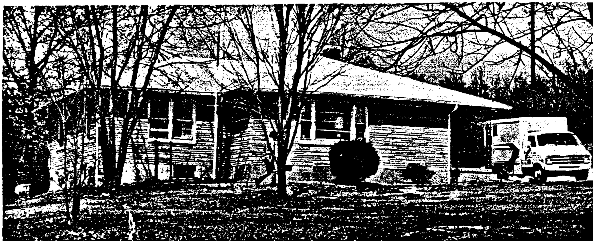
Figure 24.—Test structure 30, near a coal mine.
