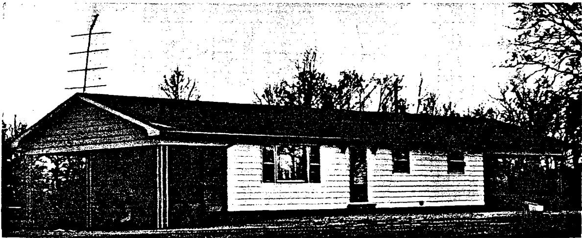
Figure 17.—Test structure 21, near a coal mine.
