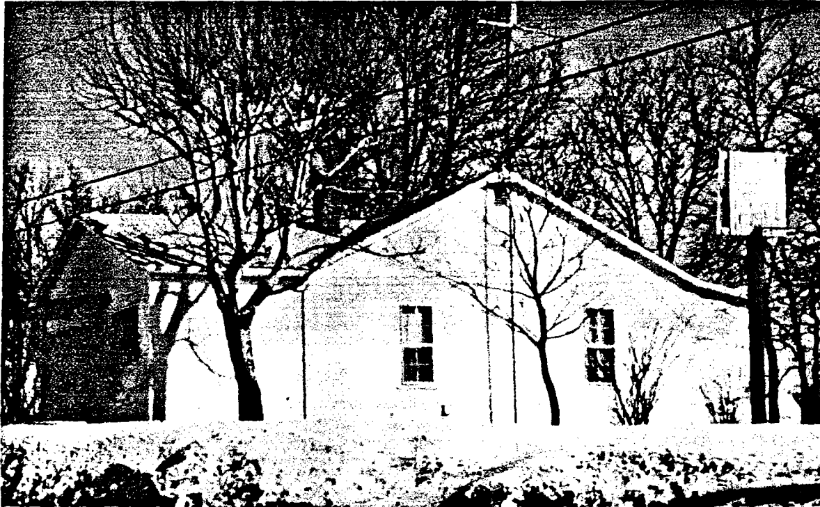
Figure 22.—Test structure 28, near a coal mine.
